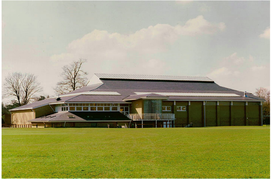
RAPID BOIL™ was installed in the Sports Centre of an Independent School in Cambridge.
