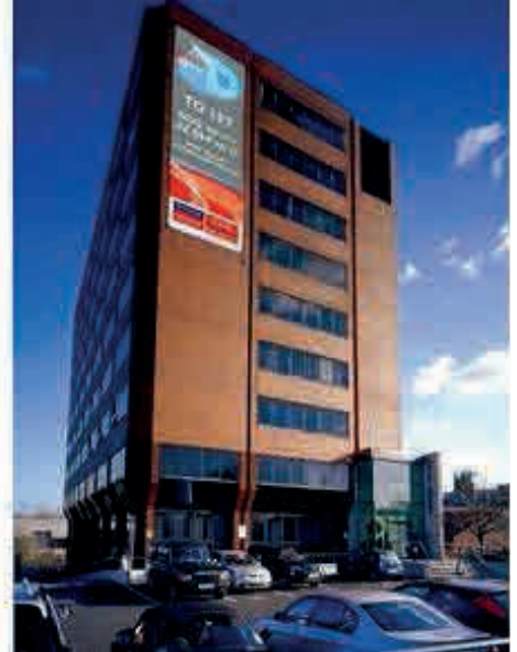
RapidBoil was installed into Dale House by Cushman & Wakefield
