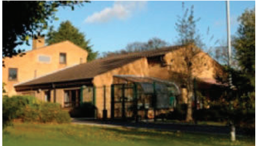
RapidBoil was installed into The Oakwood Centre, Rotherham, UK.
