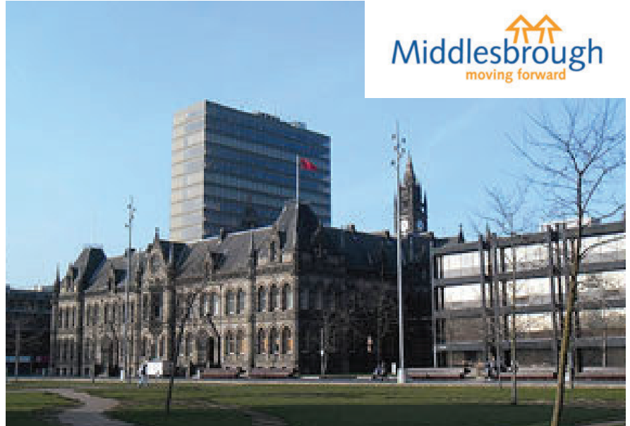
RapidBoil was installed into The Civic Centre by Middlesbrough Council
